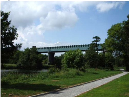
1852 Suir bridge, Caherabbey, Cahir, Co. Tipperary Railway viaduct - wrought-iron box girders on limestone masonry piers
