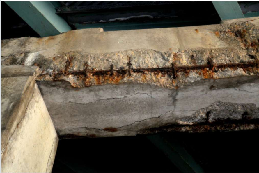
Fig 2.5.1 Arris of beam exposed by fire
