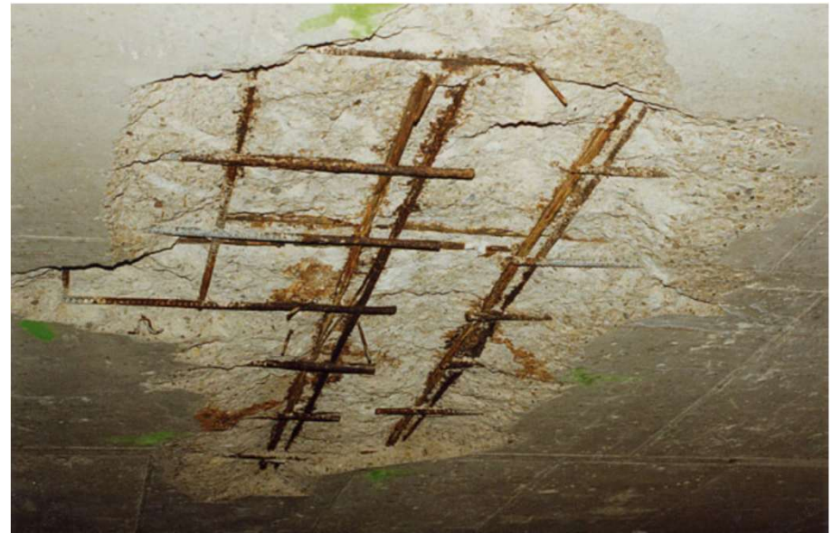
Fig 2.5.2 Soffit of slab exposed
