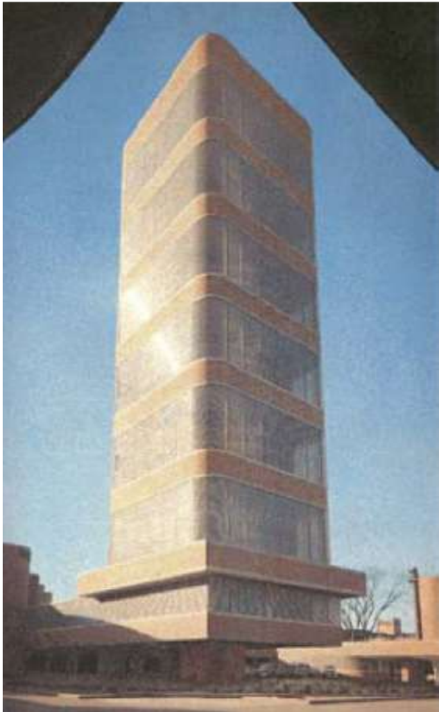
Research Tower & HQ, Johnson Wax Company, Racine, Wisconsin, 1951, Frank Lloyd Wright (National Historic Landmark) Reinforced concrete central core cantilevered from the "taproot" foundation, to resist the overturning moment caused by lateral wind loading.
