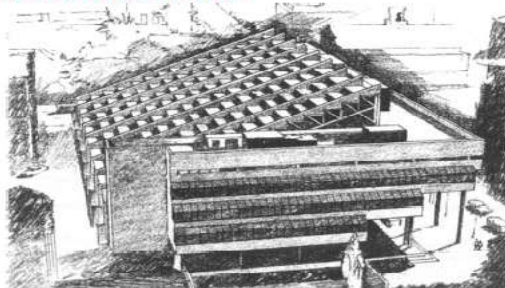
Gund Hall, (Harvard School of Design), Cambridge, MA, 1972, John Anderson, (long span truss)
